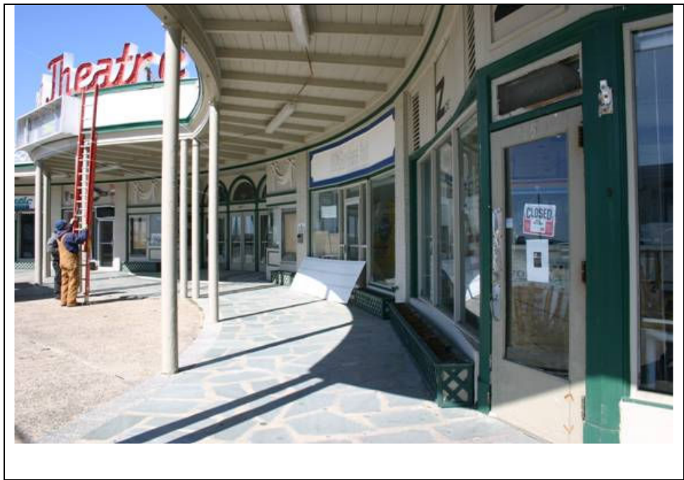
Photograph, façade (south elevation), view northwest:
